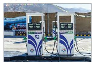
Fig. 2.2.1. Dual pump dispensing unit
