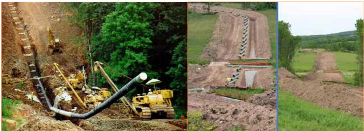
*Fig: 2.1.15 Lowering pipe into the trench*
