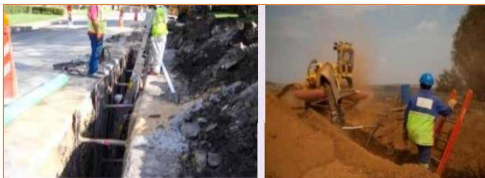
Fig: 2.1.20 prevent fall of workmen into the excavation
