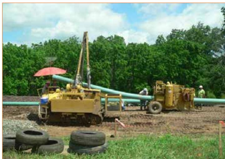
Fig: 2.1.13 Contouring or bending pipe to fit the contours of the landscape
